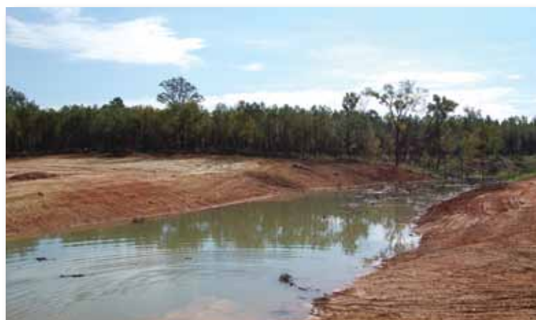
New pond/lake after construction in 2010. Will be six to eight acres in size when filled to capacity and is equipped with a well for aeration and supplemental water supply.
