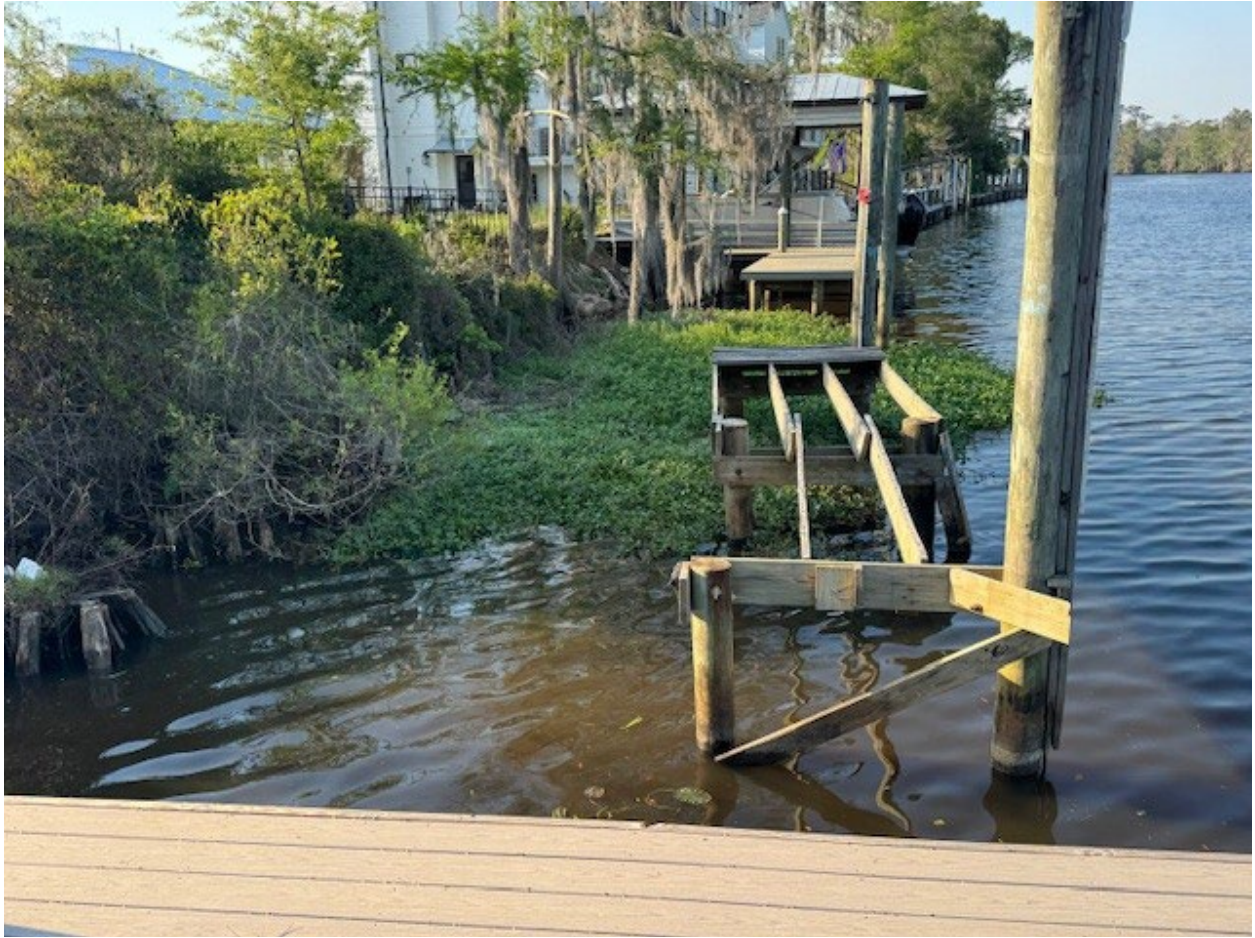
Tchefuncte River Project Location (Facing North)
