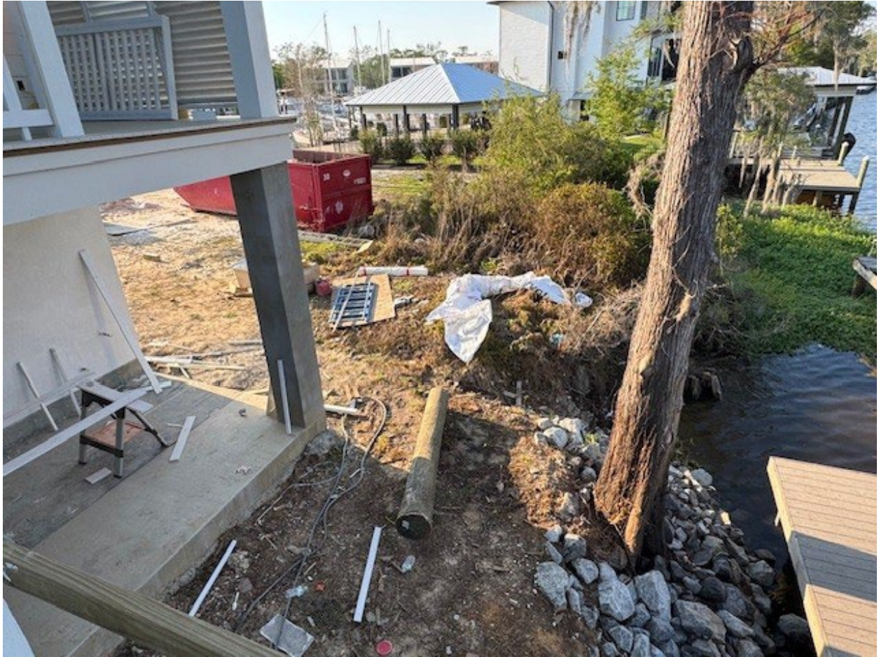
Tchefuncte River Project Location (Facing Northwest)
