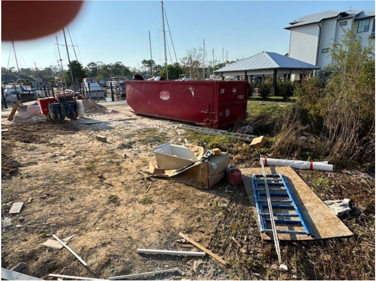
Tchefuncte River Project Location (Facing Northwest)
