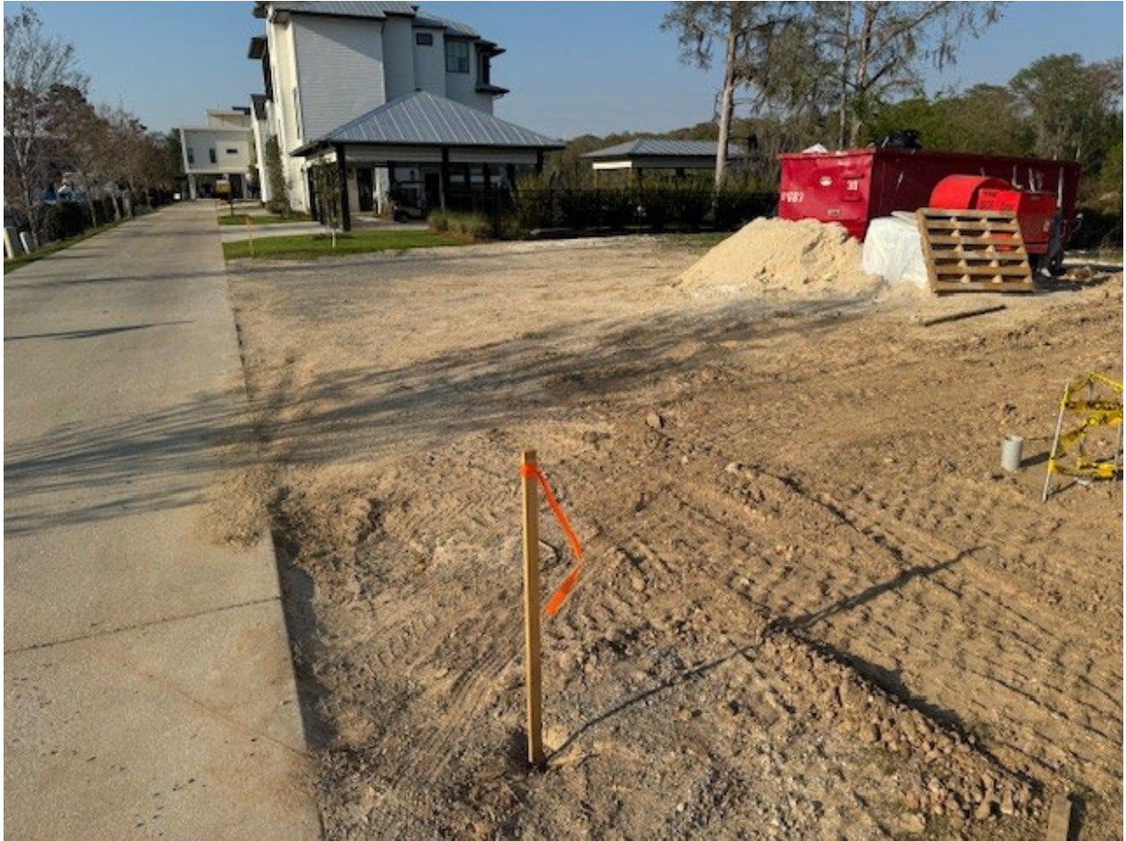
Tchefuncte River Project Location (Facing North)
