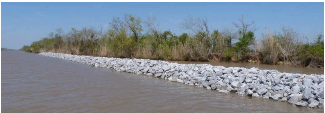
Figure 9. This photo from 2013 shows a section of the 1.5-mile rock breakwater built by Ducks Unlimited as part of a shoreline protection project along the GIWW.
