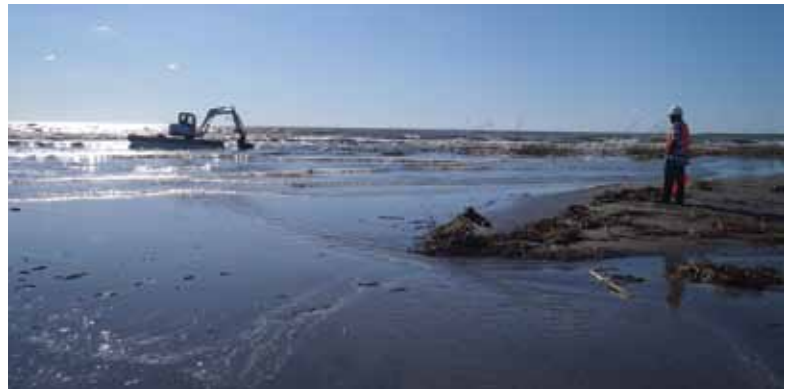
The image above is of tilling occurring within the intertidal zone of Bird Island (Pass-a-Loutre WMA) during the fall of 2011. Tilling was used in isolated areas in an attempt to remediate sediments contaminated with MC252 oil.
