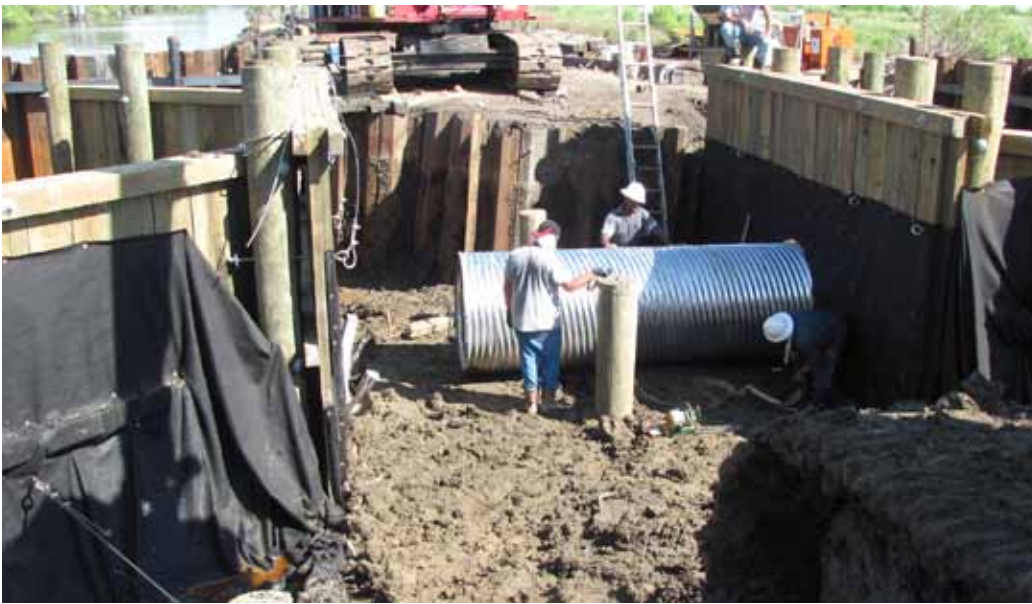
New water control structure on the St. Louis Canal for the Grand Bayou Wetland NAWCCA project.
