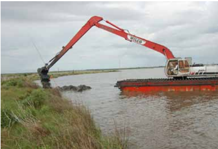
The first terrace being constructed as part of the TLCD/LDWF terrace project
