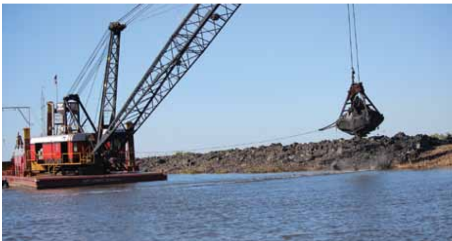
Contractor lifting levees for FEMA levee repairs at the Big Impoundment on Marsh Island Refuge.
