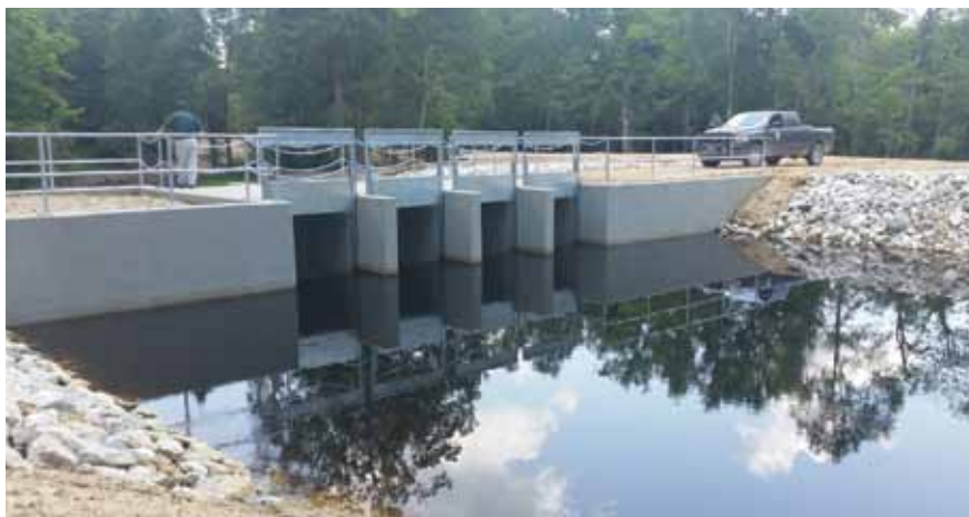
Canal gate structure at the new Dewey Wills greentree reservoir.
