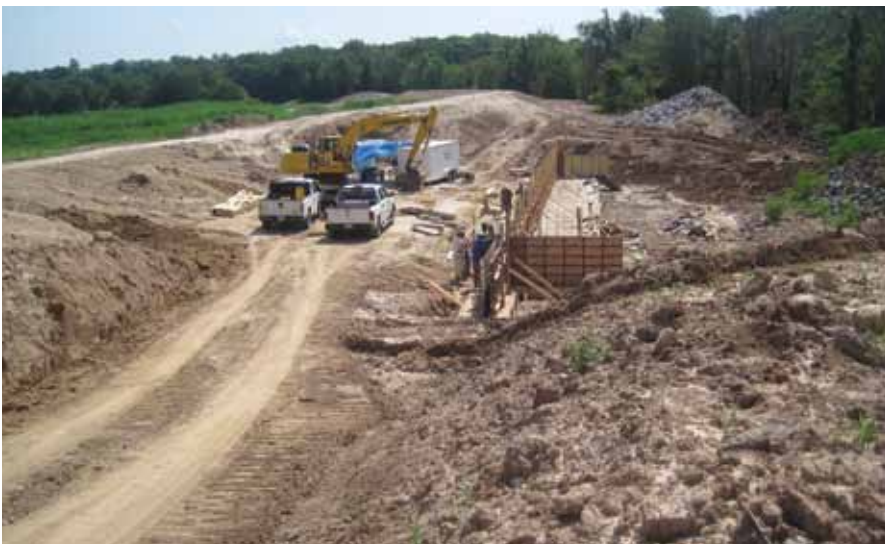
Ongoing construction of Wham Brake Water Control Structure.
