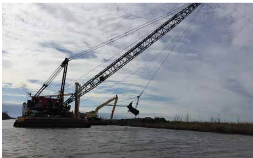
Oil operators repairing levees.
