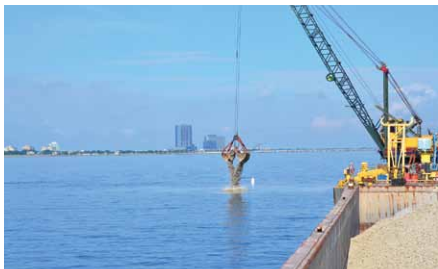
Crushed limestone and recycled concrete are deployed at the West End reef site in Lake Pontchartrain. The reef site was created in conjunction with planned renovation of the boat launch and new fishing pier facilities.
