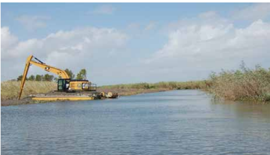
Excavator constructing a new crevasse on Johnson's Pass at Pass-a-Loutre WMA.
