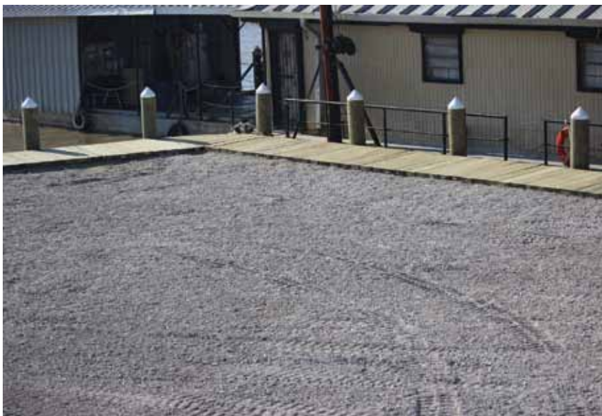
New bulkhead and dock at State Wildlife Refuge.
