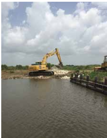
LEFT: Contractor adding rip rap to a water control structure at Pointe-aux-Chenes WMA to prevent scouring. RIGHT: One of the water control structures at Pointe-aux-Chenes WMA that was blasted and painted to prolong life of structure.
