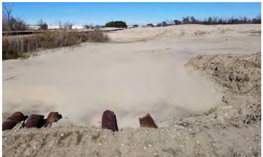
Commercial dredge pit in St. Bernard Parish pumped full of water bottom sediment dredged from the Mississippi River
