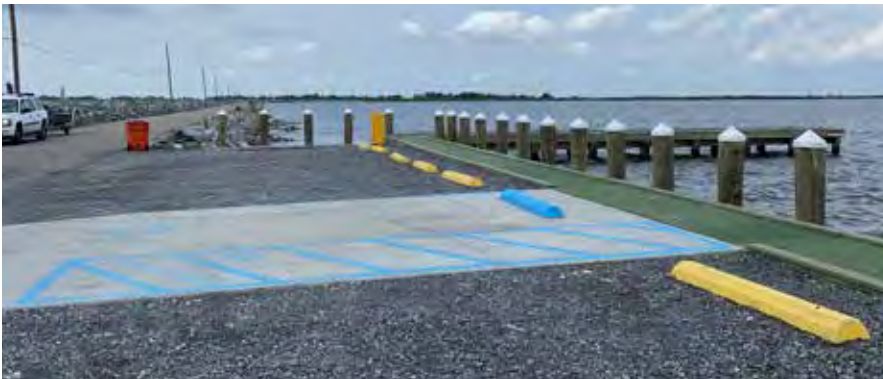
Pointe-aux-Chenes WMA pier construction.
