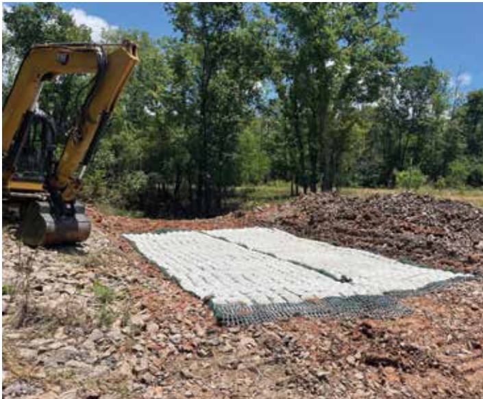
LEFT: Loggy Bayou WMA - GTR Spillway mats installation RIGHT: Bodcau WMA - dove field prep
