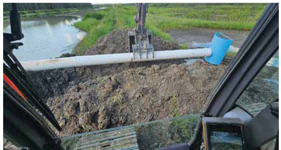
Sherburne South Farm WCS replacement
