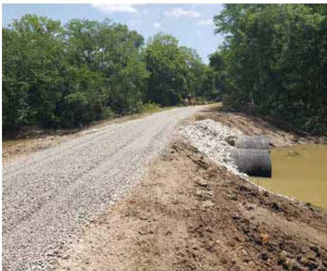
LEFT: Richard K. Yancey WMA Routen Camp culvert replacement RIGHT: Richard K. Yancey WMA Warren Trail culvert replacement
