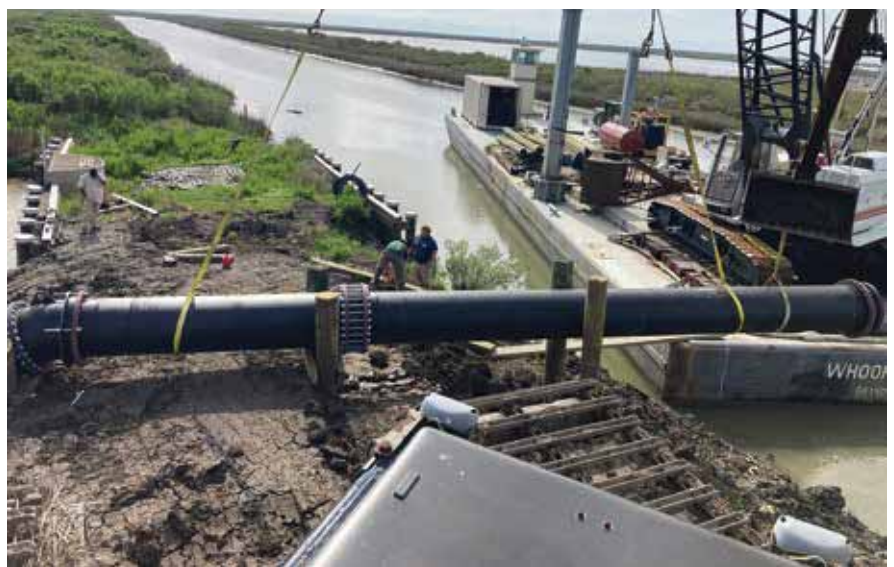
Unit 3 pump installation
