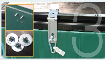
**3** Attach the hasp and latch plate to bottom lip and lid of can. Each component is secured by placing bolts through pilot holes and securing with washers and locking nuts.
