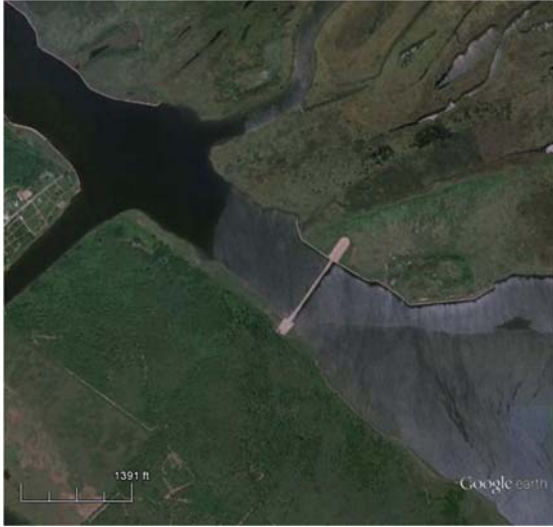
Figure 2. MRGO rock dam.
