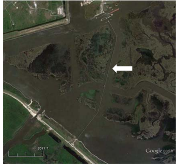
Figure 3. Storm surge protection wall at Bayou Bienvenue.
