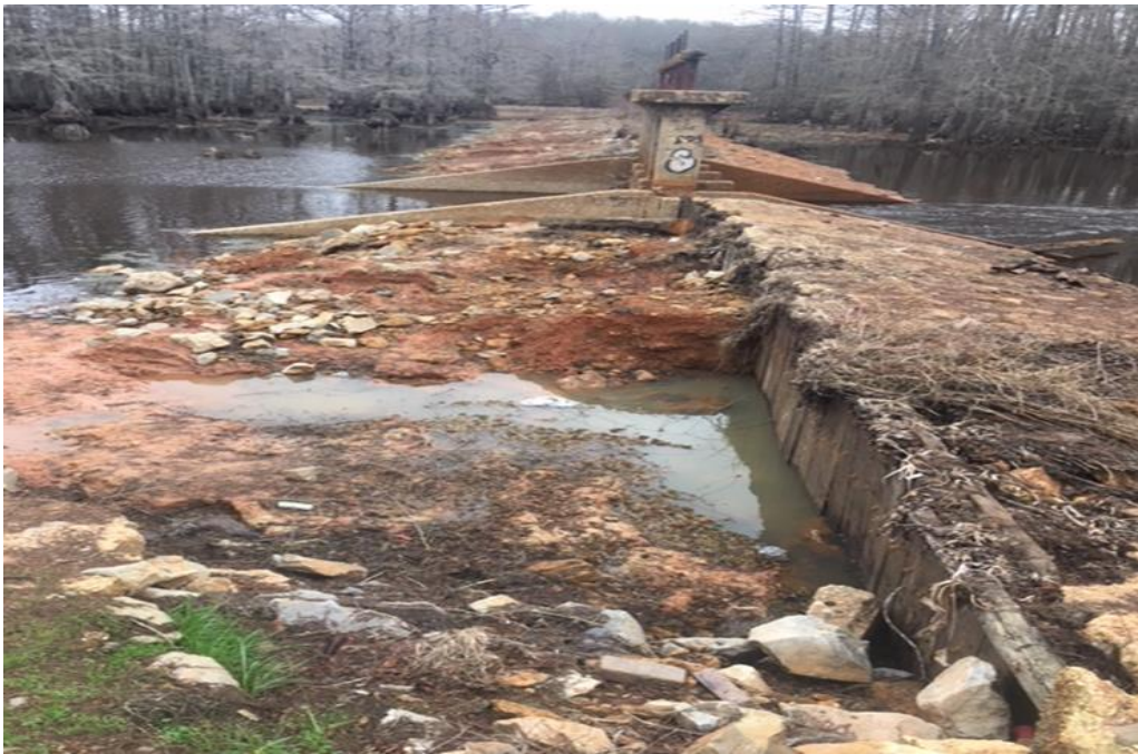
Figure 1. Clear-Smithport Lake Spillway showing severe erosion along face of the spillway following the 2016 floods.
