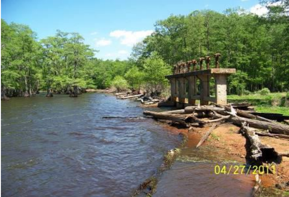
Figure 2. Smithport Lake Dam control structure
