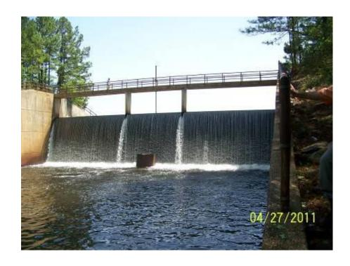
Water level (MSL) -176.5 MSL at normal pool stage. Normal seasonal water level fluctuations from approximately 175 MSL to 178 MSL
