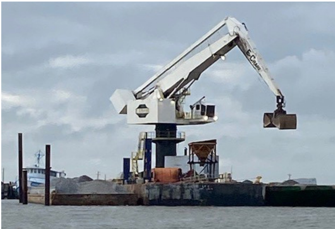
CRANE PLACING LIMESTONE FOR THE CONSTRUCTION OF THE 2023 CALCASIEU LAKE CULTCH PLANT.
