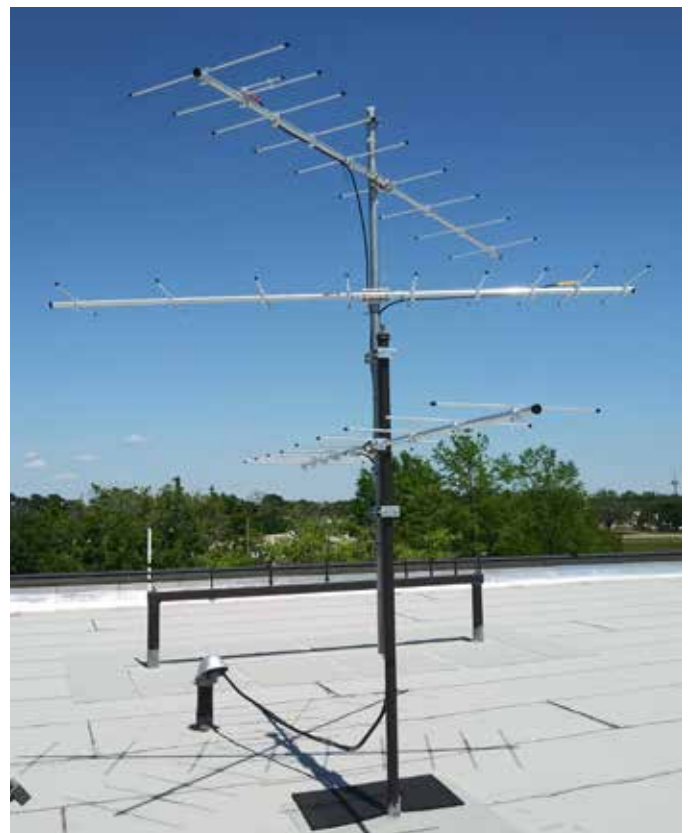
Motus Wildlife Tracking System (Motus): A temporary VHF tower used for the Motus Wildlife Tracking System at Richard K. Yancy Wildlife Management Area (ABOVE). A VHF station, with antennas mounted on the Lafayette LDWF office building rooftop, used for the Motus Wildlife Tracking System (BELOW).
